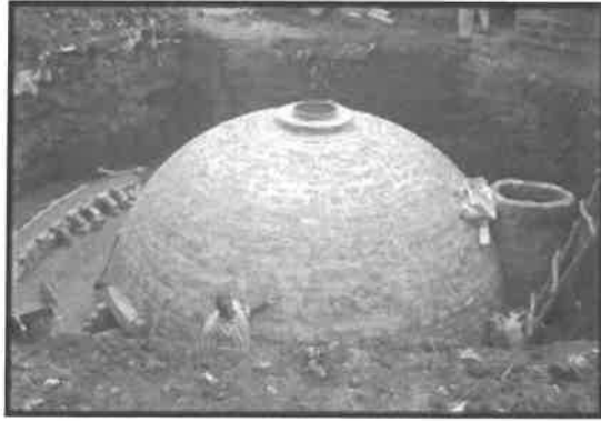
Figure 1 Completed Biogester Dome
